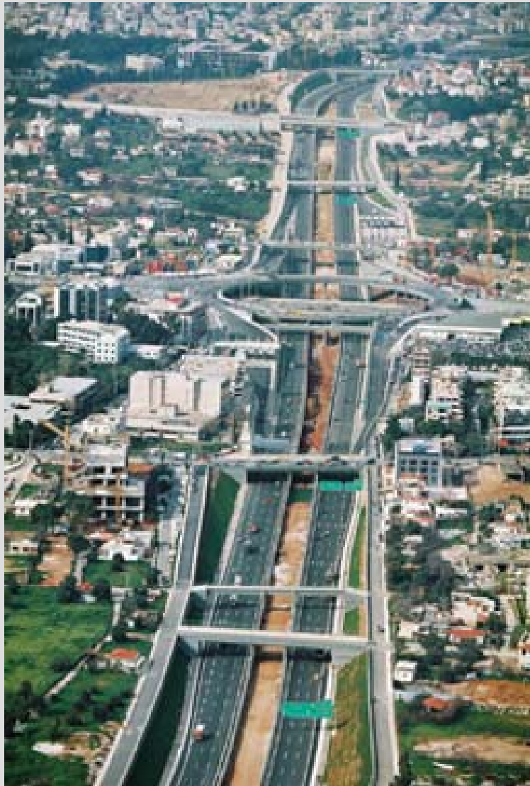
Attica Tollway, Greece
