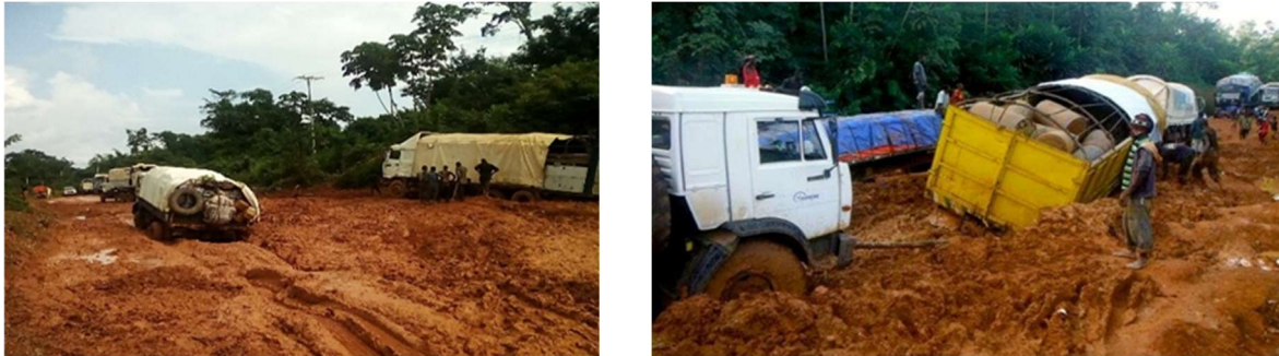
Figure 11: Typical condition of critical sections under truck loading in the rainy season
