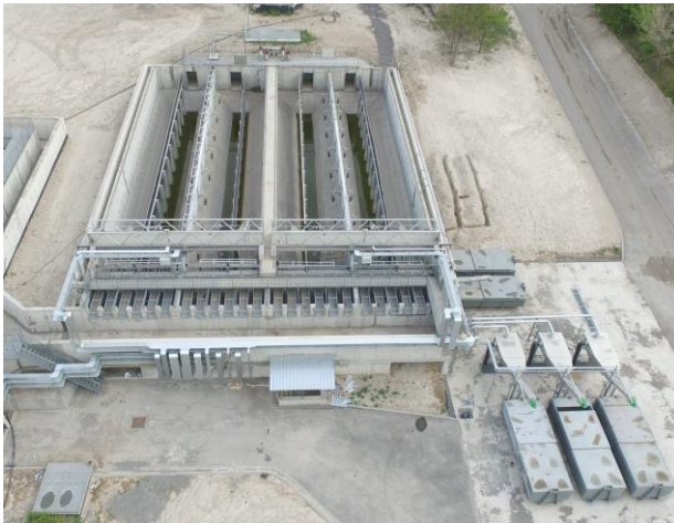
Figure 15: the new wastewater treatment plant in Yerevan (source Veolia, with permission)
