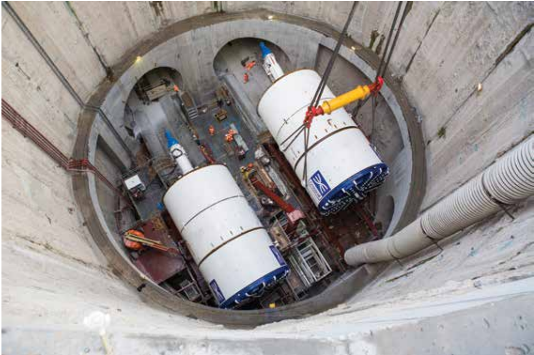
IMAGE 11.4. Tunnel Boring Machine Victoria Being Lowered into the Launch Shaft
