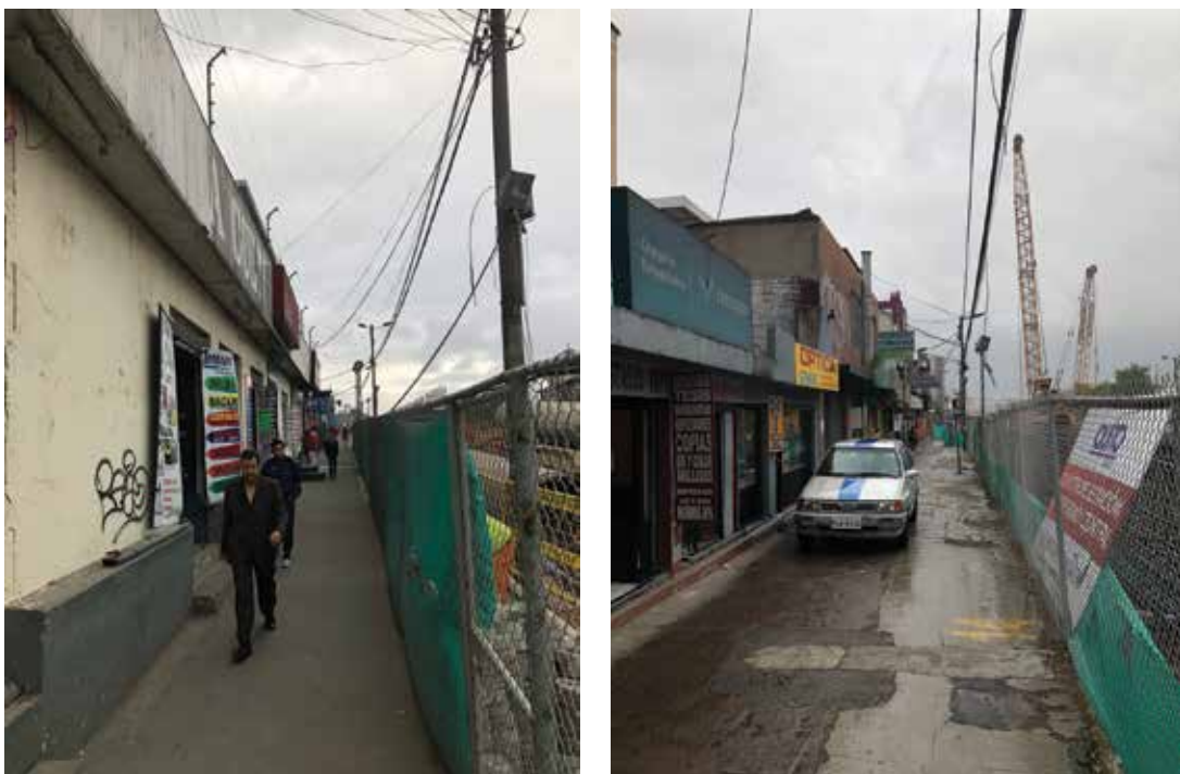
IMAGE 14.1. Residence and Business Access during Construction: Quito Metro, Ecuador
