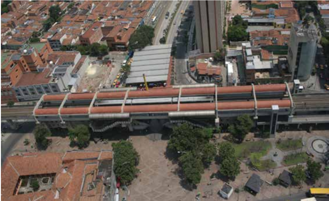
IMAGE 14.3. Downtown Station Integrating Brick Materials, Colors, and Texture to Minimize Visual Impact and Increase Compatibility with Existing Architecture: Metro de Medellín, Colombia
