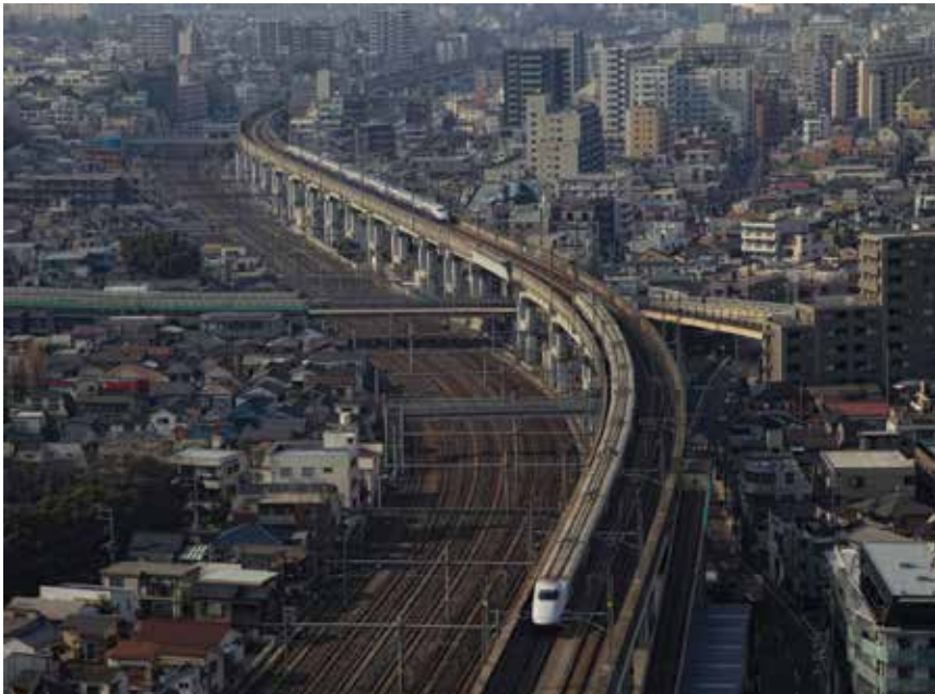
IMAGE 11.1. Elevated Intercity High-Speed Rail and At-Grade Urban Rail Lines, Crossed by a Highway Overpass and Pedestrian Flyover: Tokyo, Japan
