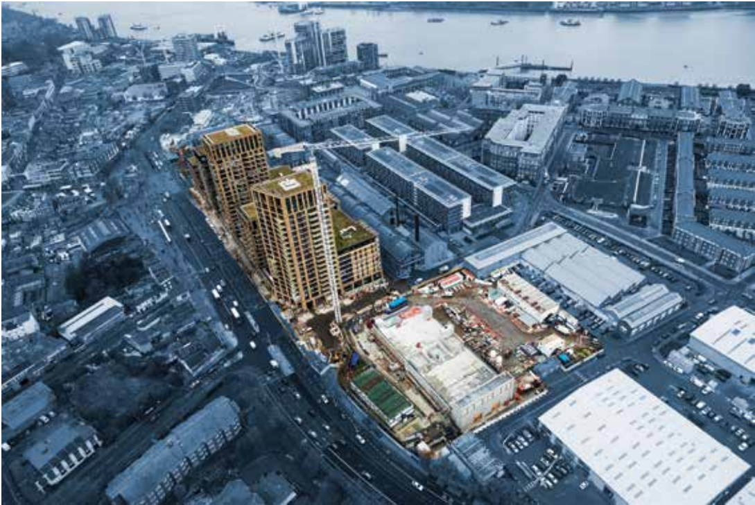
IMAGE 16.7. Aerial View of Woolwich Station with Berkeley Homes Oversight Developments: London, United Kingdom
