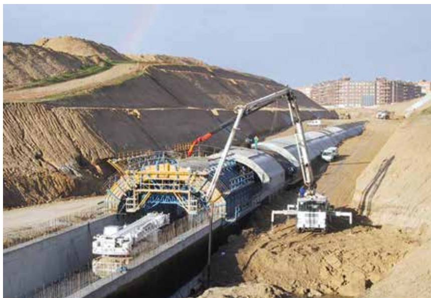
IMAGE 11.6. Construction of an In-Situ Tunnel on Line 12 Metro Sur: Madrid, Spain
