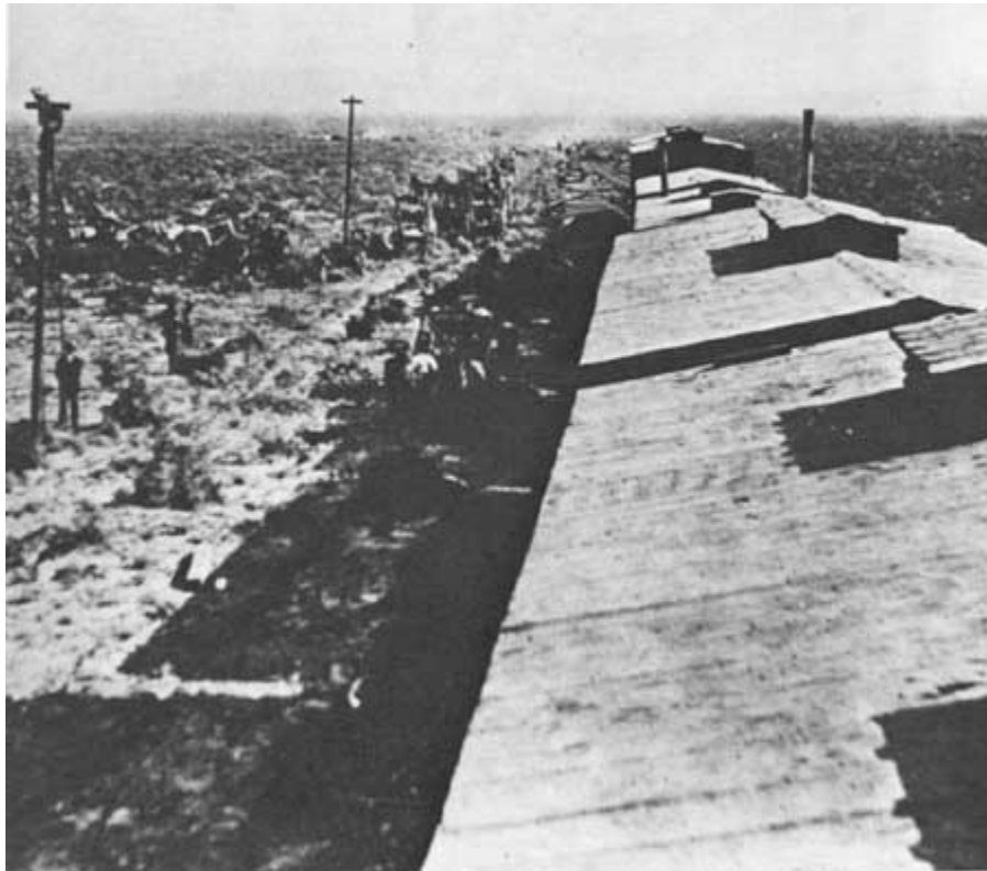
Figure 8.50: Installing the telegraph lines on poles along the railway
