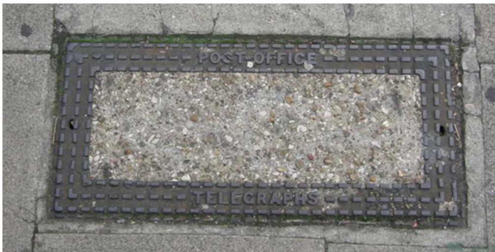
Figure 8.6: Access cover for buried telegraph cable in the United Kingdom
