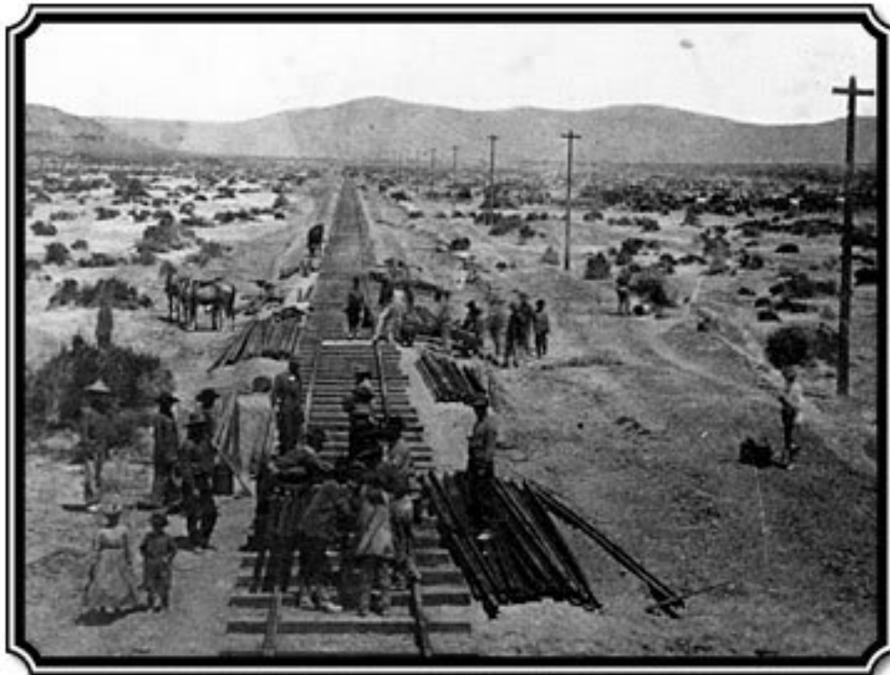
Figure 8.49: Simultaneous construction of transcontinental railroad and adjacent telegraph poles in 1868 293
