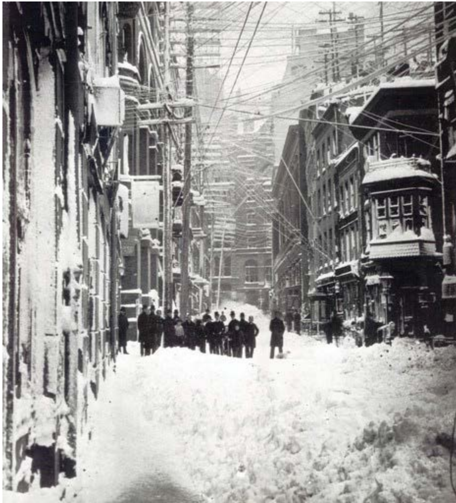
Figure 8.52: New York City ordered burying of electric and telecom wiring after the Great Blizzard of 1888
