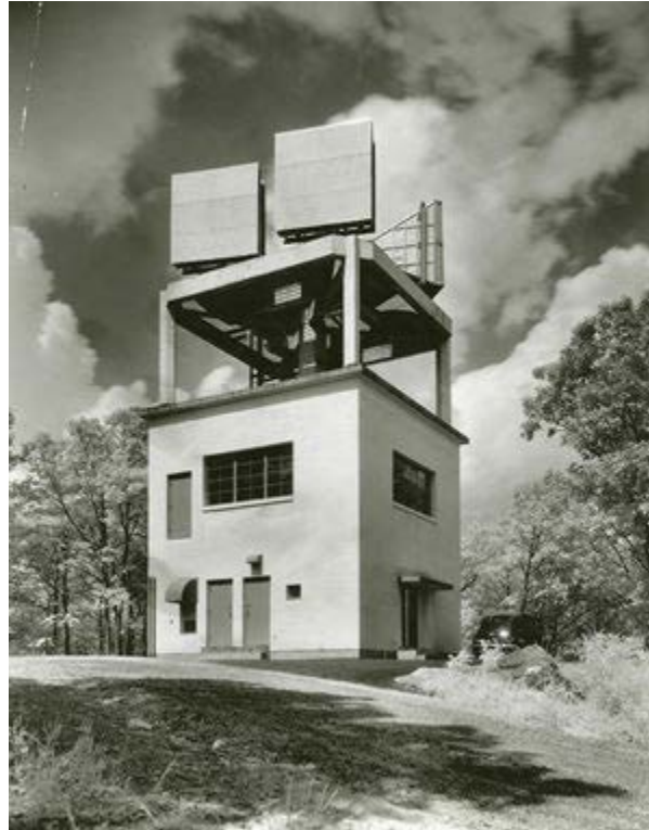
Figure 8.10: Microwave tower used in first commercial long distance telephone relay system
