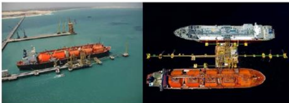
Figure 18 Example of onshore regasification terminals
