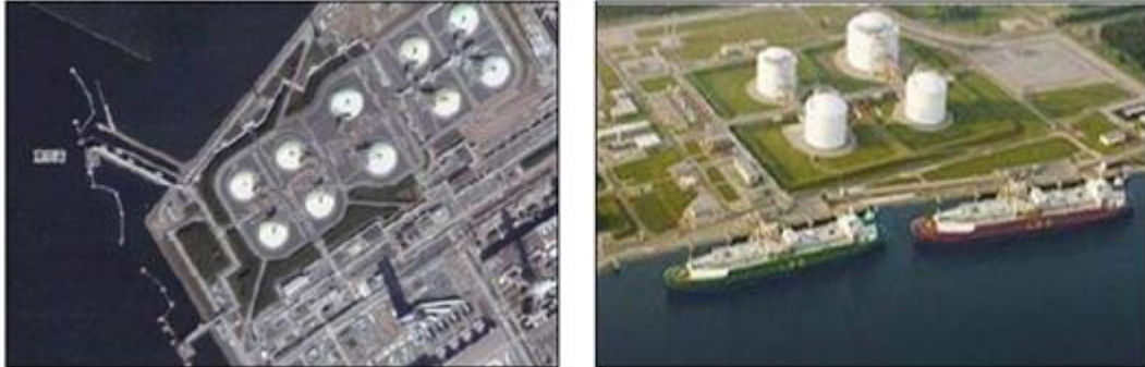
Figure 17 Example of onshore regasification terminals
