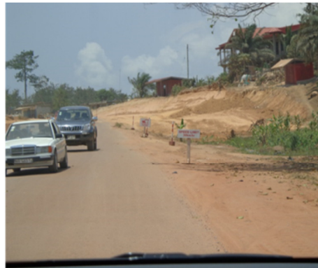
Current works at Kanwosorado Rd.
