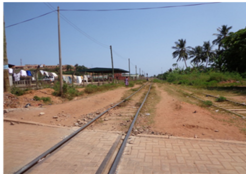
Rail Road existing right of way
