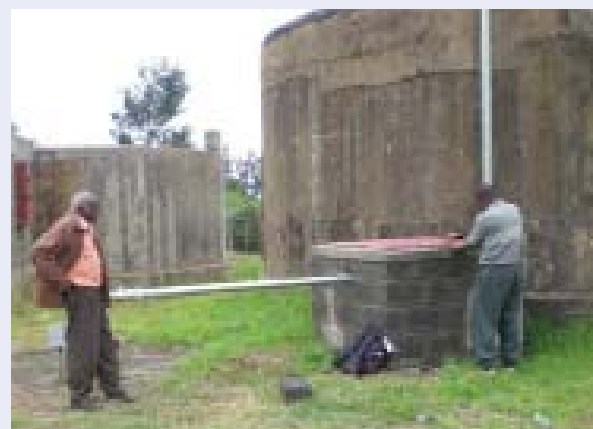
Storage and distribution tanks at Karaweti Water Project in Githunguri division of Kiambu district. The community borrowed $50,000 from K-Rep Bank to develop a new source and install meters for all its customers. As a result, revenue collection increased by 90% and the reliability of water services increased tremendously, with 87 percent of customers receiving water seven days a week, up from 8 percent before the investment.
