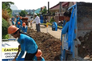
Laid about 273km of pipes
