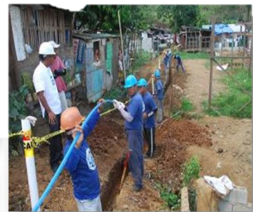
Replaced 52km of pipe mains
